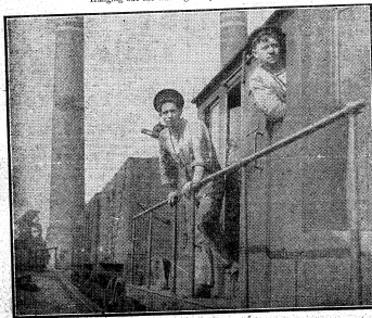
Naval ratings at work at the Southern Railway's power station at Wimbledon. Through-out the strike they have fully demonstrated "Jack's" ability.
