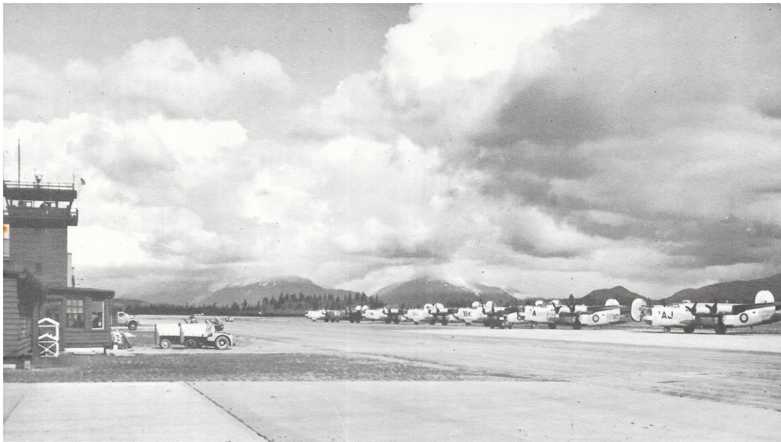
Control Tower, outside.
